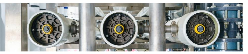
The first-pass system typically uses seawater RO membranes because they can handle the higher pressures needed to overcome the high osmotic pressure caused by the high salt content. The permeate from the first pass then goes to the second-pass RO, using either seawater or brackish water RO membranes.
